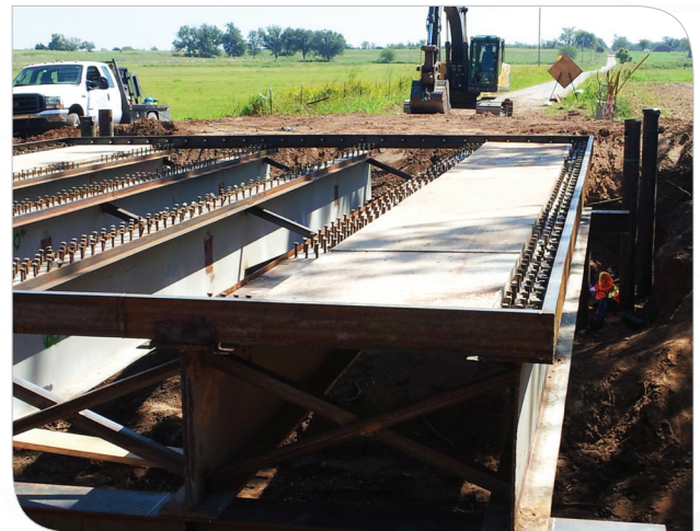
Recycled beams from the I-40 Crosstown Expressway are being used to refurbish over 350 county bridges across Oklahoma including this one in rural McClain County. (photo courtesy of Association of County Commissioners of Oklahoma)
